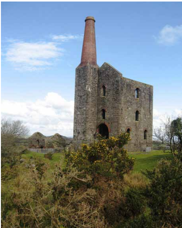
Prince of Wales engine house, South Phoenix Mine © Mike Scott
